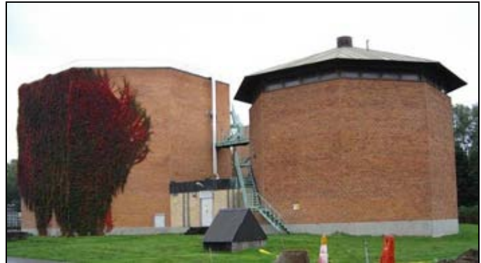
Figure 7 Anaerobic Digesters in Kristianstad, Sweden
