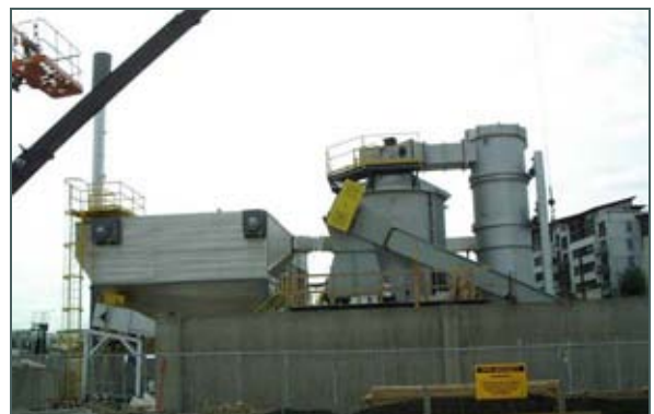
Figure 8 Dockside Green Gasification Plant Under Construction, August, 2008
