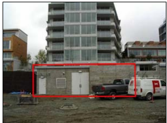
Figure 5 Dockside Green wastewater treatment plant, May 2008
